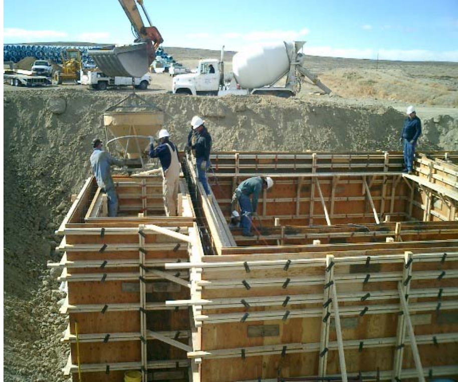
Figure 7. District Construction Crew Placing Concrete at Hidden Valley Pipeline Inlet Structure
